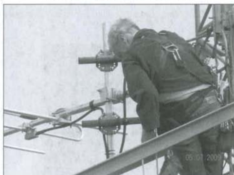
WA1ZMS 2m beacon antenna – FM07FM
